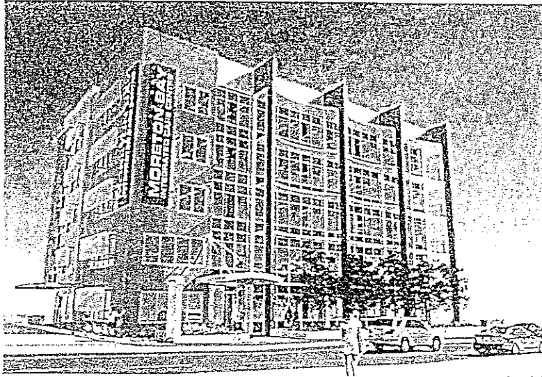
Building Frontage to Anzac Avenue
